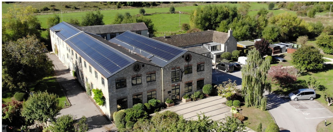
Our head office in Witney has 125 solar panels.
